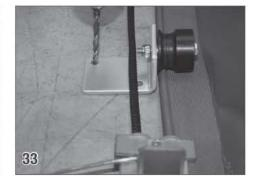
To help the cover roll up evenly, install a cover roller 2-3 inches behind the guide feed. Secure the cover roller to the deck using the screws (15) and anchors (25) provided.
