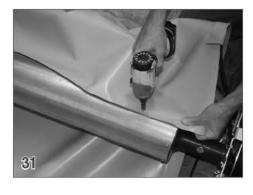
The first two screws need to be 3" from the end of the tube. Distribute the slack of the cover evenly across the length of the tube. Secure the cover to the roll-up tube using tek screws every 2-3ft. When attaching the cover to the tube, do not use folds or pleats.
