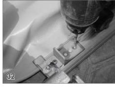
Install a guide stop on the end of the guide near the mechanism to keep the cover from retracting too far. Secure the stop to the deck using the screws (15) and anchors (25) provided. Run the key switch in the uncover position to roll the cover up on the roll-up tube. Check the cover to be sure it rolls up evenly.
