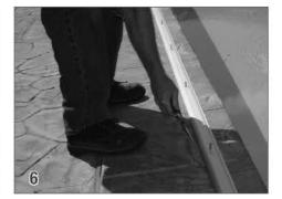
Feed the rope into the back channel then pull the rope down the back side of the guide toward the cover housing.
