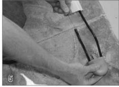
Feed the rope through the pulley assembly (17) and insert the pulley housing into the end of the guide.
