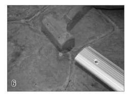
At one end, use a rubber mallet to tap the guide sections together.
