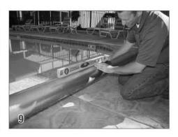
With the mechanism and tube assembled, check the roll-up tube for level. This is crucial for a properly operating cover. Adjust the non motor end as needed to level the roll-up tube.
