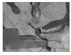
Use the 1 1/2 hex head screws (26) and anchors (25) provided to secure the motor end and non motor end to the deck.
