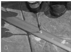
Complete the fastening of all guide screws flush to the top of the guide. Clean concrete dust from guides and pulley endcap. Make sure ALL screws are flush with the top of the guides.
