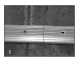
The two sections of guide should be tight together.
