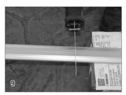
Cut the guide to the proper length on both sides of the pool. Note: Always wear safety goggles when using powered equipment.
